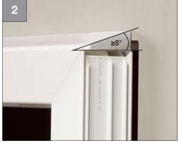
Suggestion: Mount a wedge for better water discharge ≥5°. Observe the manufacturer's specification
