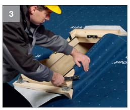
Secure the roof underlay membrane to installation and skylight frame on all sides
