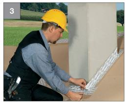
• Starting at the bottom and working upwards: repeat on each side
