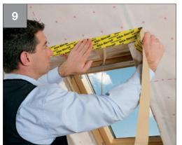
Finally seal the overlaps using Sicrall 60
