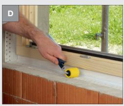
Press the tape on firmly with a roller to ensure even more protection
