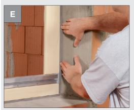
Fill joint seam with insulation material without cavities
