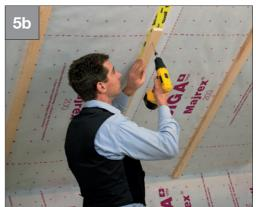
For wide joists or extremely high insulation material weight we recommend installation of the membrane in the direction of the rafters, sealing in the rafter area and longitudinal installation of the battens
