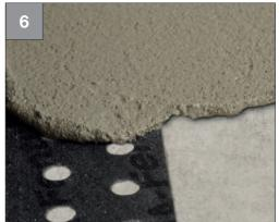
The width of the substrate to be plastered covered by Fentrim must not exceed 60 mm without counting the Fentrim perforated zone.
