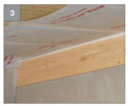
Unfold Corvum and mount vapour control layer
